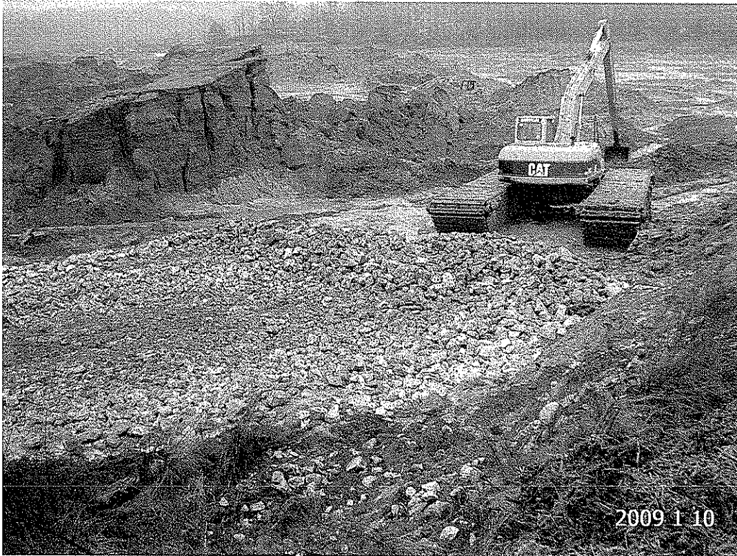
Photo 3: Rip Rap Being Placed After Lunch
