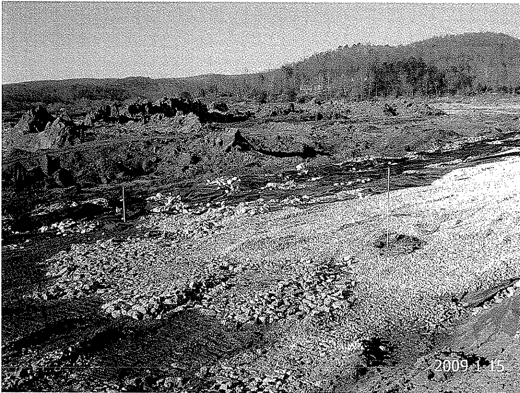
Photo 1: PZ-1 and PZ-2 At South End Stabilization Area (Looking North)
