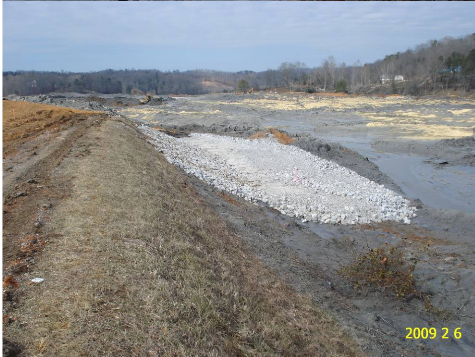
Figure 8. Dike C Wraparound Before (top, looking east) and During (bottom, looking west) Armoring
