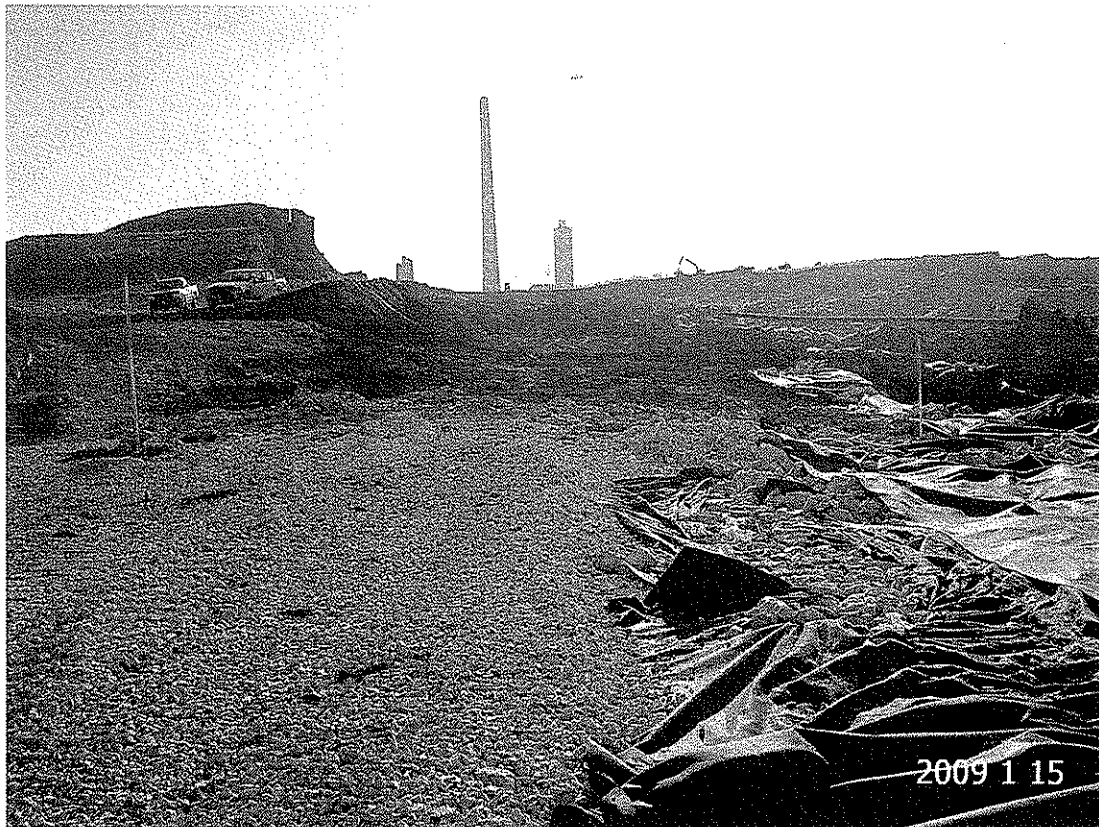
Photo 4: PZ-1 And PZ-2 At South End Stabilization Area (Looking South)
