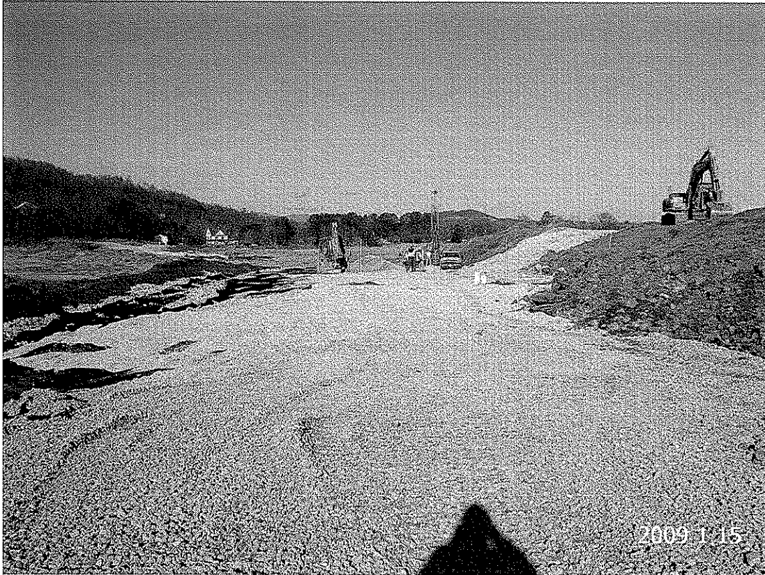
Photo 5: PZ-5 And PZ-6 In Stabilization Area (Looking North)
